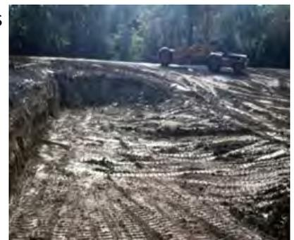
bulldozer and two earth-moving pans on the site. Within about a week he had the hole dug out. It was 12-foot-high at the north end and ground level at the south end.
